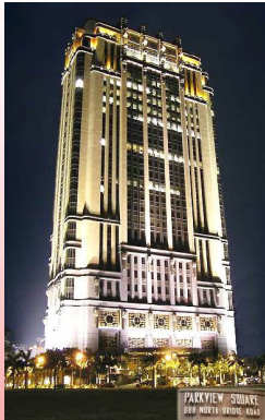
PARKVIEW SQUARE 300 NORTH BRIDGE ROAD
